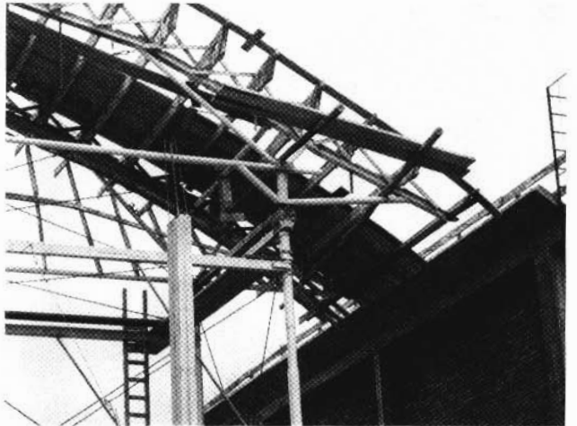
fig. 229: Detail of a device to allow movement of the formwork past the tie-rods. Two parallel metal beams, separated by wood blocks, are placed in the direction of the horizontal movement, between the pipe column and the upper lattice truss.
